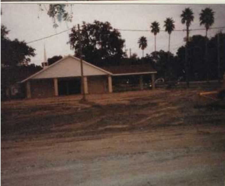
October, 1986 - The final touches are being applied. The building will soon be ready for our first worship service.
